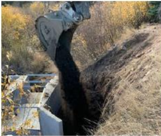
Placing backfill around flume
