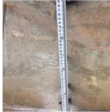
Installed staff gauge
