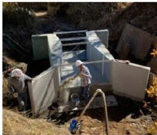
Final touch-ups on flume concrete
