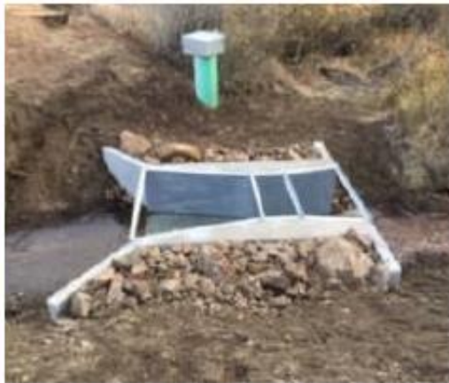
Completed flume installation
