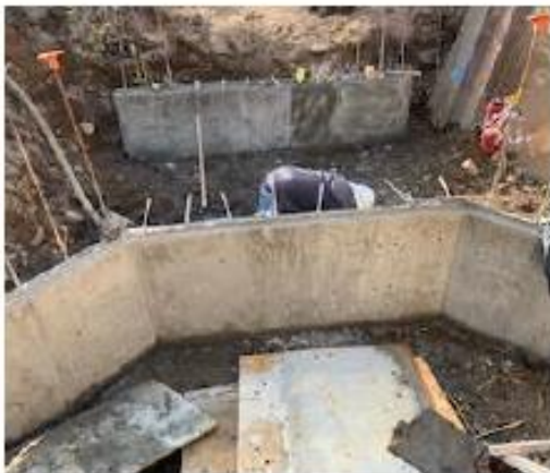
Removing forms for footers
