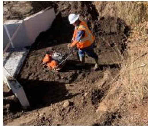
Compacting backfill
