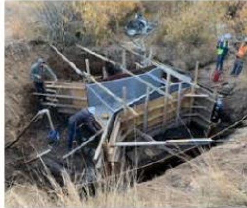
Installing rebar and forming
