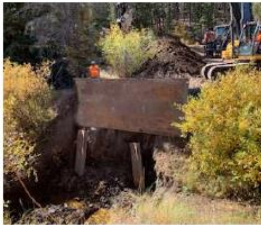
Installing steel plates
