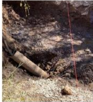
Placing rock for sump
