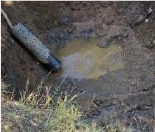
Construction of sump
