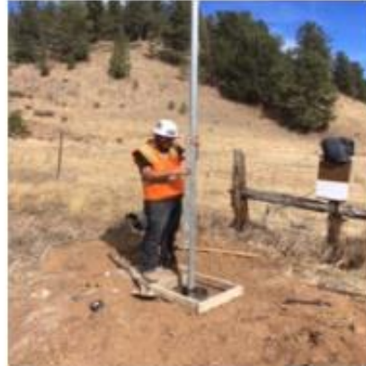
Installing 2" mast pipe
