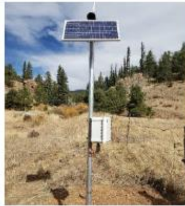
Completed mast with solar panel and equipment
