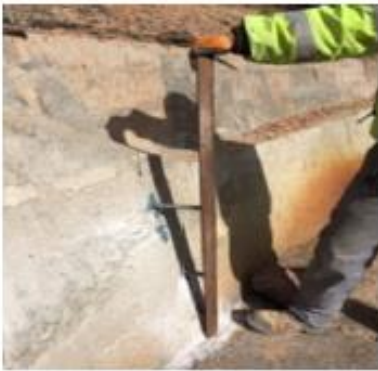
Installing support for staff gauge
