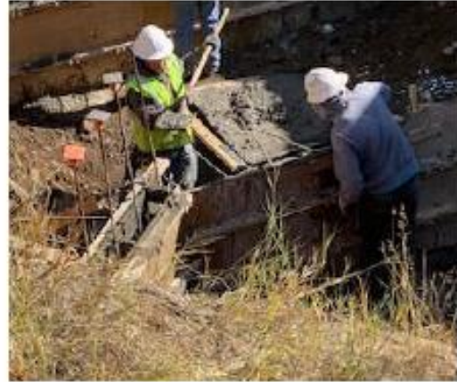
Placing concrete for footers
