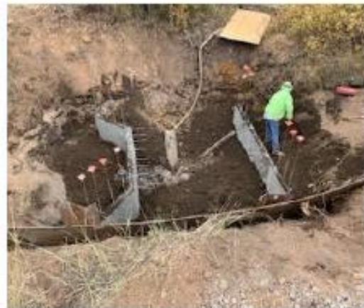
Placing fill around footers
