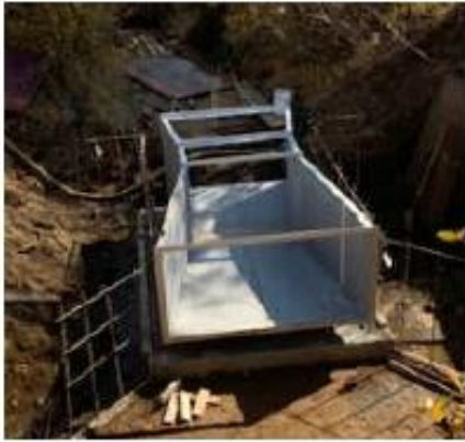
Installing rebar and forming
