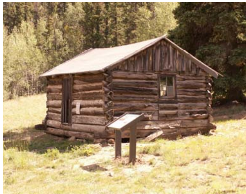
The Derby Cabin prior to restoration in June 2011.
